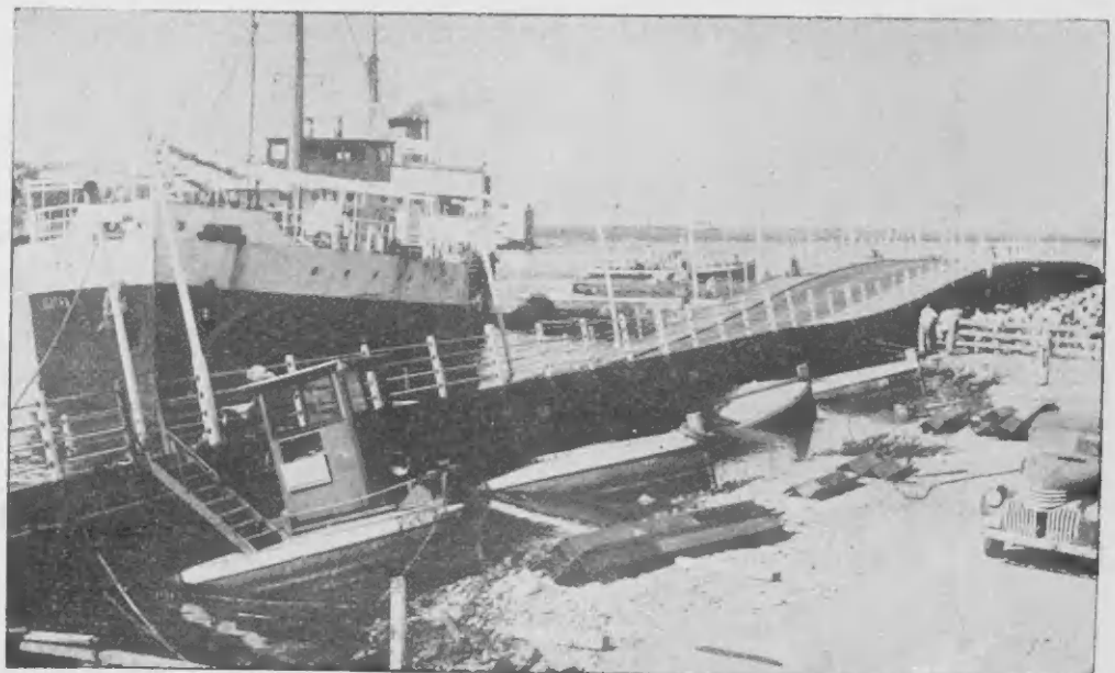
Curaçao's famous pontoon bridge across St. Anna Bay was seriously damaged July 6 when a tanker smashed into it. Nine of the pontoons sank and it will be sometime before the bridge is repaired. Meanwhile, the people of Willemstad cross from one side of the city to the other by means of launches. The accident occurred when the strong currents of the bay drove the tanker toward Fort Amsterdam; trying to avoid a collision, the tanker turned its wheel sharply and ran into the bridge.
